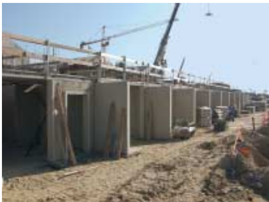
Figs. 14 and 15 Residential building.
